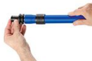
3. Push the fitting into the expanded pipe
